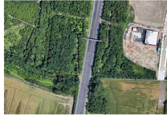
Existing aerial photograph of M11 bridge
