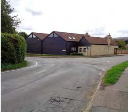
Existing photograph of Coton High Street - Cambridge Road Junction
