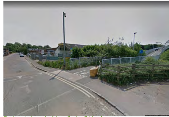
Existing photograph of Jane Coston Bridge Approach, Junction with Cambridge Road
