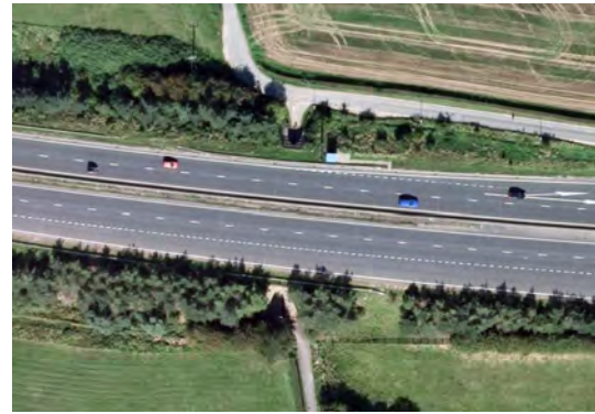
Existing aerial photograph of A14 Underpass
