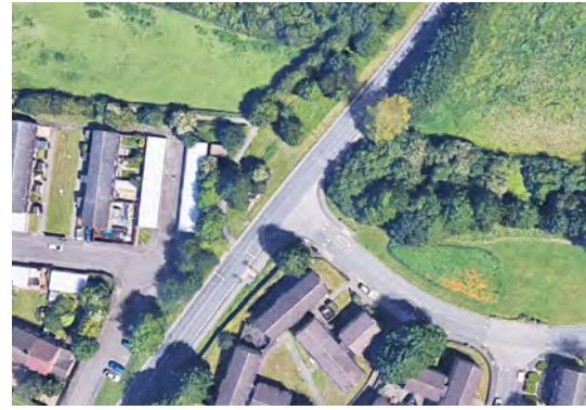
Existing photograph of Ditton Lane Underpass
