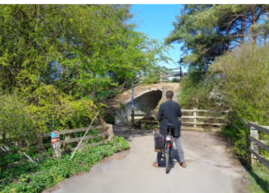
Existing photograph of Southern Approach to A14 Underpass along Private Road
