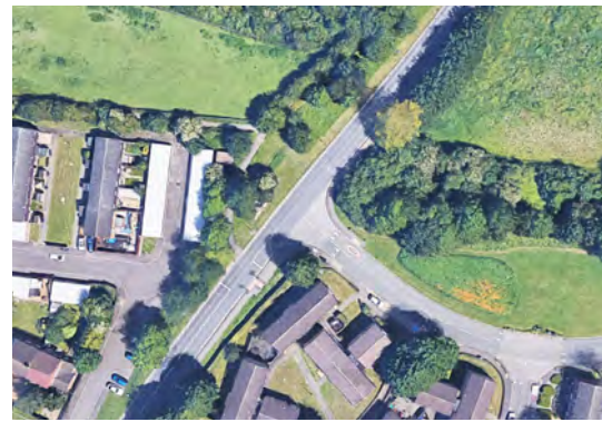
Existing photograph of Raised Table to Fison Road
