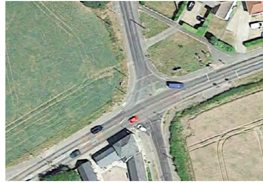
Existing photograph of Quy Road Crossing at Anglesey Abbey
