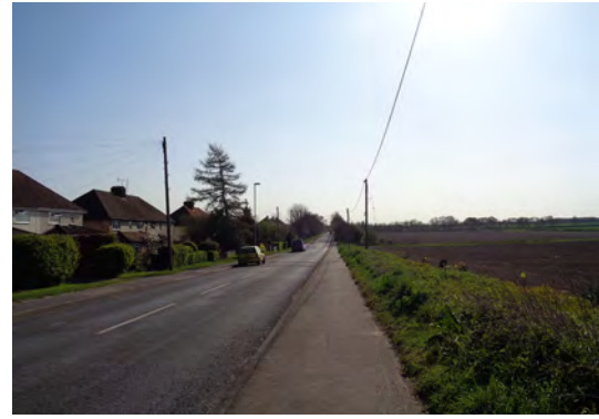
Existing photograph of Shared Surface Path Parallel to Bell Road
