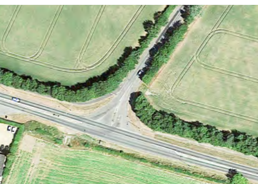
Existing photograph of Bell Road Junction with Newmarket Road, A1303
