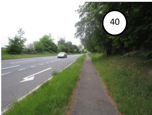
A new bridge could span between the raised land behind the trees to the left of the photo and connect with a new ramp in place of this existing highway path. Details would need to be agreed.
